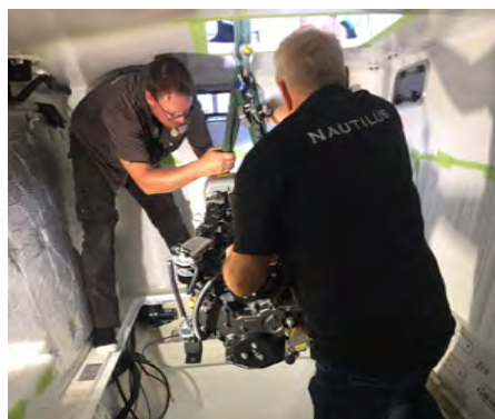
The Yanmars being installed in MV Comfortably Numb
