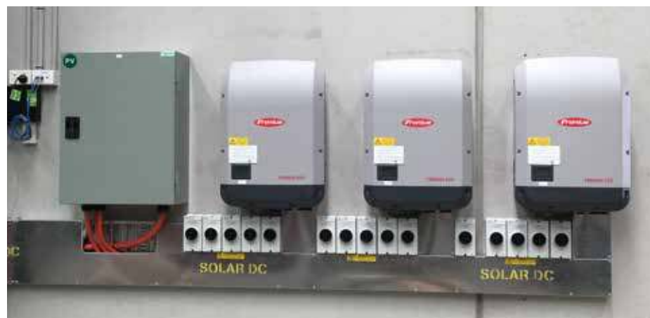
Three AC inverters are located in the Melbourne's warehouse
