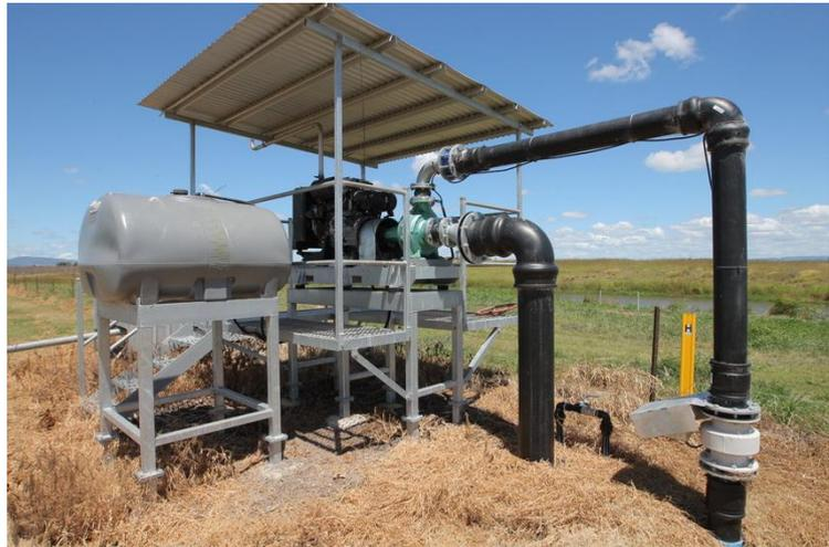
With the Hermitage Research Facility located alongside the Swan Creek, the Yanmar driven pump has been installed to pump water from the creek to an off-stream storage dam. When in use it involves pumping water over a 2000 m run and at the same time lifting it 20m up the hill into the dam.
